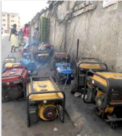
○ Diesel-powered electricity generation Nigeria 1
